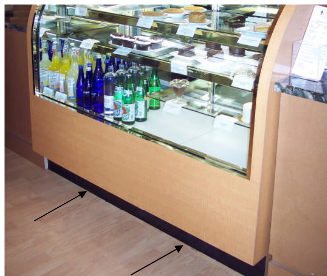
Silicone Bead Permanently Sealing Display Case to Floor. Case Must be Sealed on All Sides.
